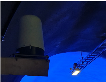
Ryfast Tunnel, Norway 102 radar installed Across 28.8km
