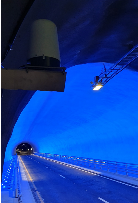
Ryfast Tunnel, Norway 102 radar installed Across 28.8km
