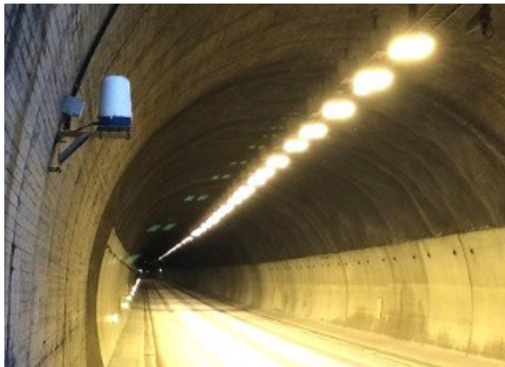
Bergeland Tunnel, Norway: 3 radar installed across 700m
