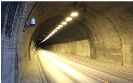
Bergeland Tunnel, Norway 3 radar installed Across 700m
